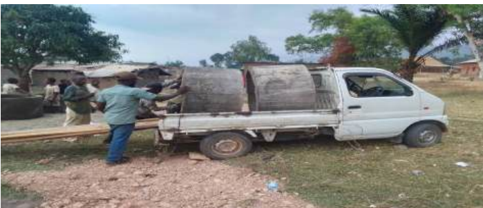
Figure 4 : transport of concrete buse to Kakombe site
