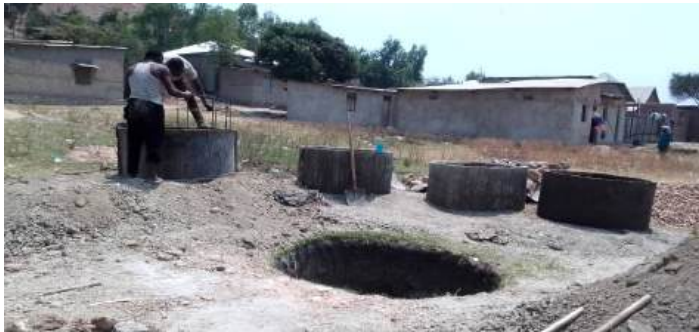
Figure : making of cylindrical casings to stabilize the well
